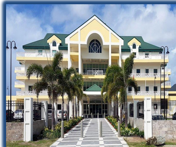
New Government Administration building of Sint Maarten
