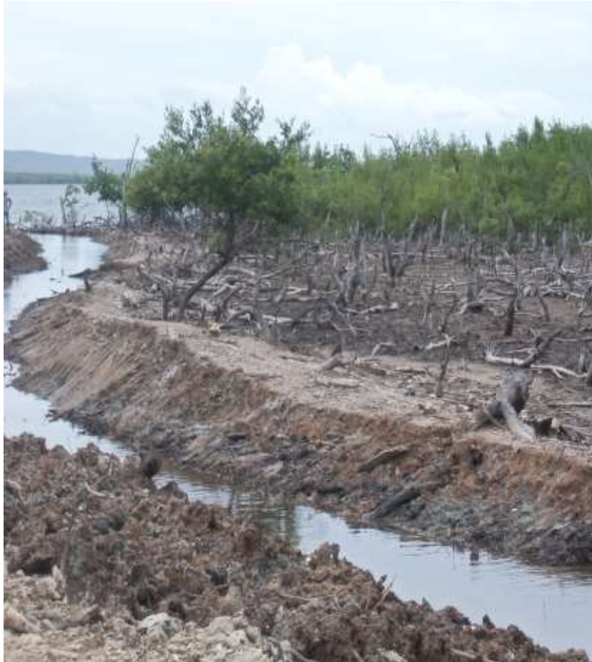
Building Hydrological Channel- Portland Cottage
