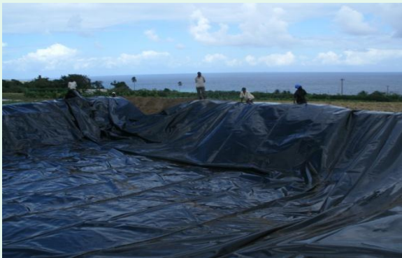
Putting lining in place
