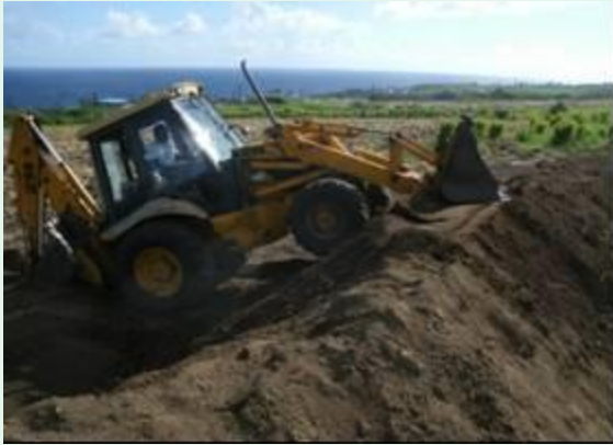
Initiation of excavation Works
