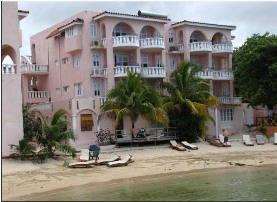
Figure 4.6.1: Coastal Tourism Development Vulnerable to Storm Surge and Sea Level Rise
