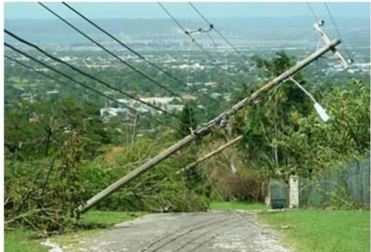
Figure 9: Hurricane Dean Impacts on public utilities in Jamaica
