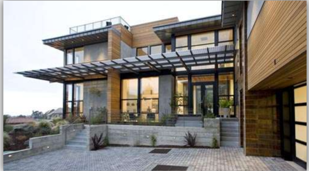
Margarido House - McDonald Construction & Development, Inc. California.
