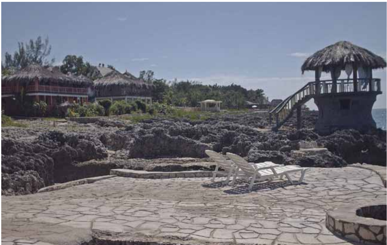
Hotel infrastructure built close to the shoreline and the cliff edge is highly vulnerable to storm surges and wind damage associated with hurricanes
