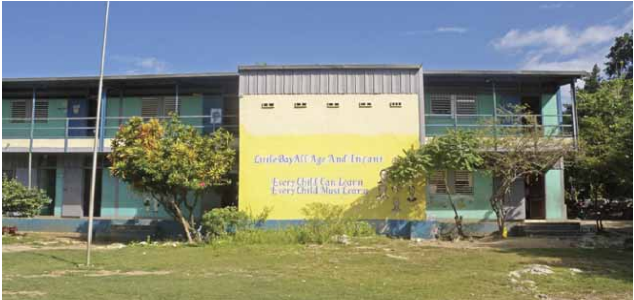
The All Age School at Little Bay is used as a storm shelter
