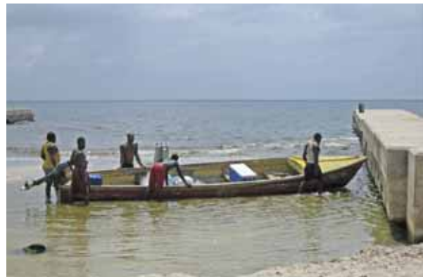
Concrete groynes on Long Bay beach are used to trap sand and prevent the long shore drift of sediment, but they can result in sediment starvation of down-current sections of the beach
