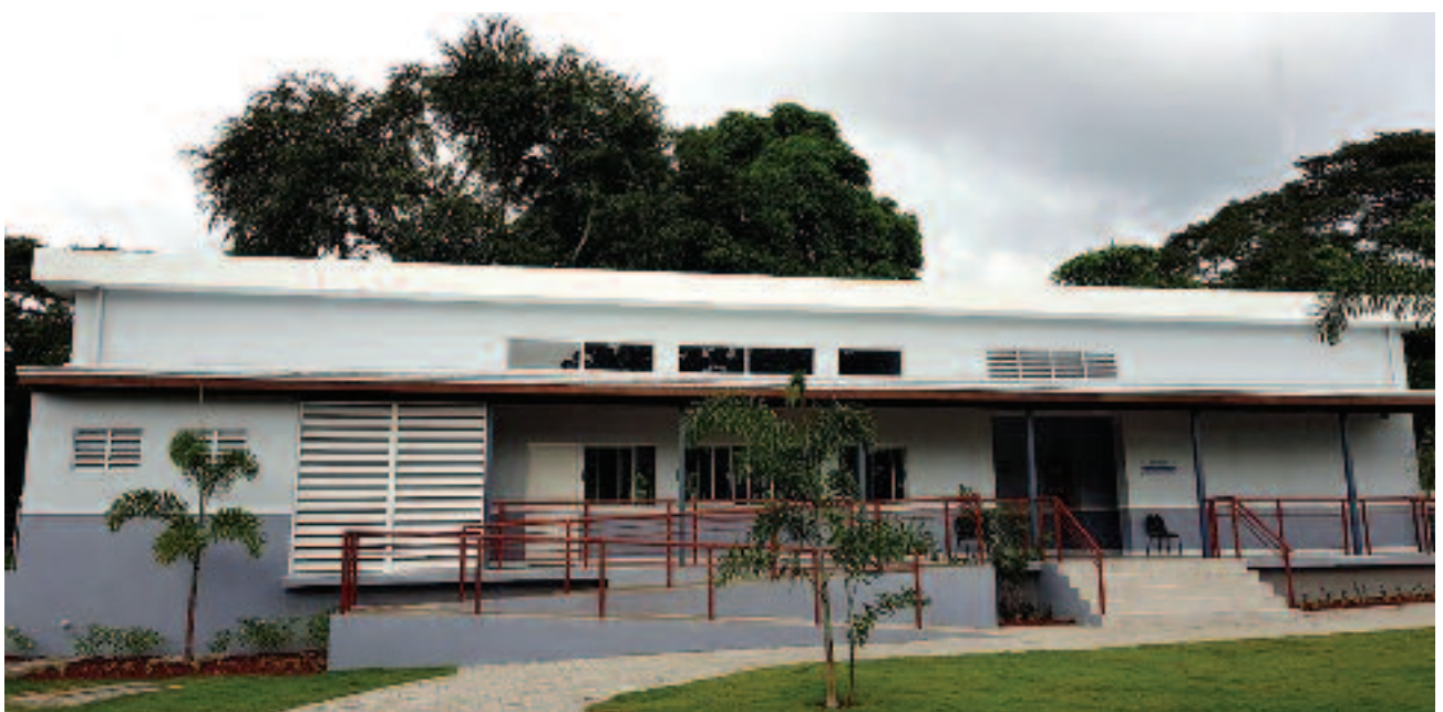
Official Opening of the Net-Zero Energy Building, October 2017
